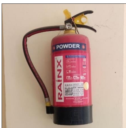
Figure 9: ABC-MAP 90 type Fire Extinguisher installed at each floor of the campus building
